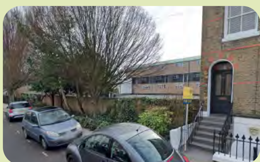
3. Existing site from Spencer Rise
